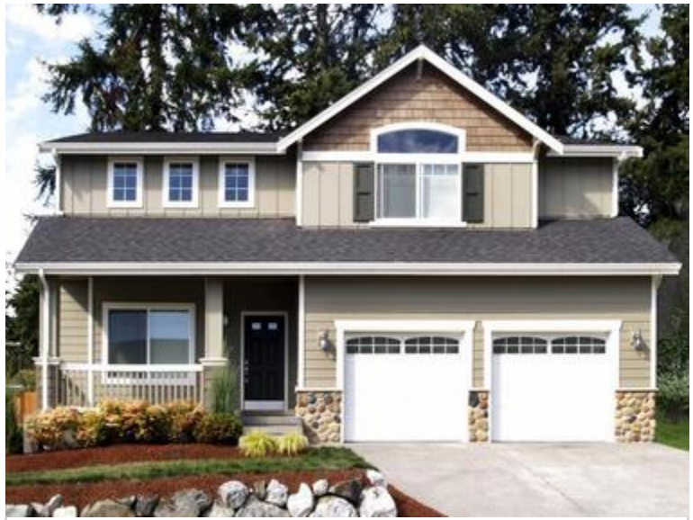
Simulated windows change an ordinary garage door into one with more curb appeal. | Classic Coach House Accents/Lacks Enterprises
